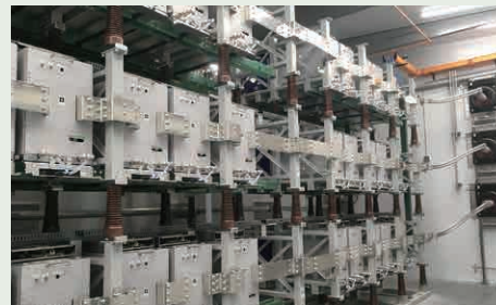
•Static Synchronous Compensator
